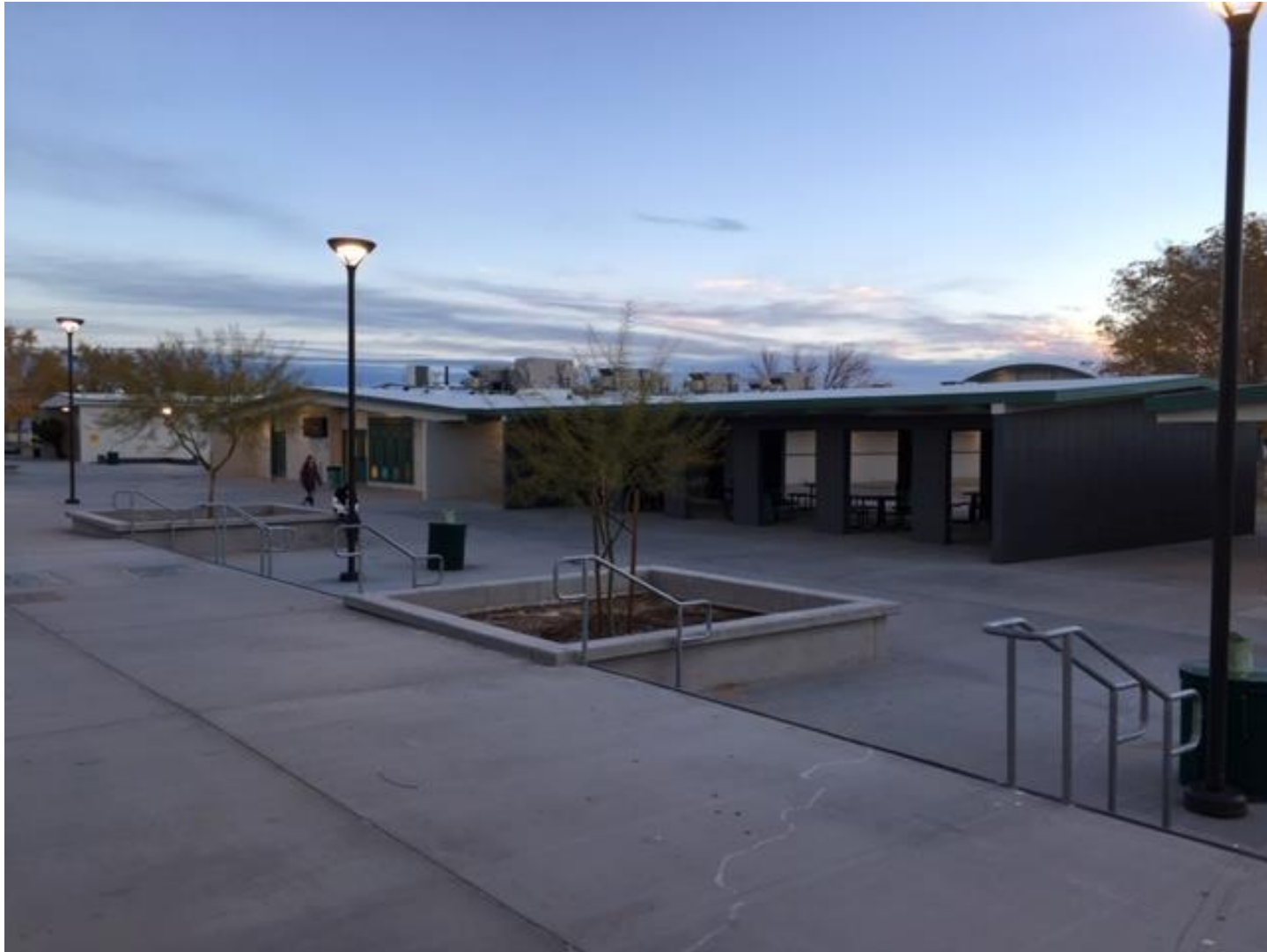
Central Courtyard and New Lunch Shelter Remodeled and ADA Accessible
